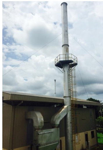
A bio-mass boiler for reducing the company's carbon footprint.
